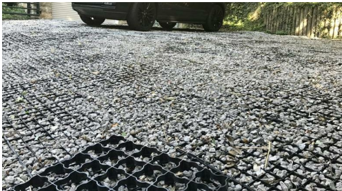
Figure 3: Ecoraster installation example
