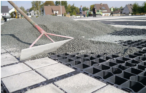
Figure 2: Ecoraster installation example
